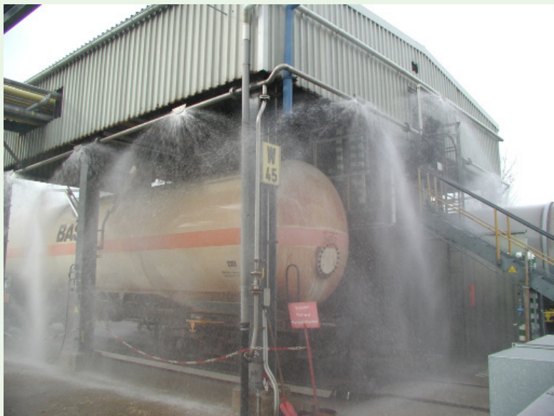
Figure 23 The water curtain system in action. The sprayed water builds a closed curtain
