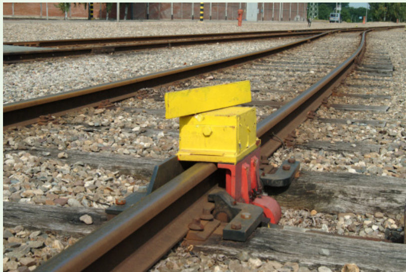
Figure 17 Derailment devices to prevent other RTCs from entering the loading/unloading station
