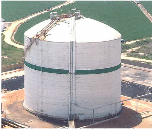
Picture 3 Single steel wall tank with earth dyke
