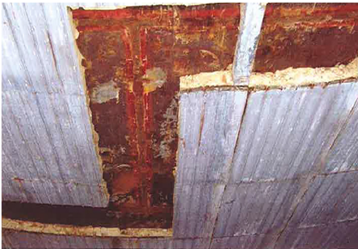
Picture 8 Weld area to be inspected, with insulation removed
