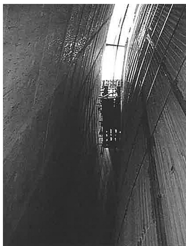
Picture 7 Inspection of the tank from the outside in the annular space
